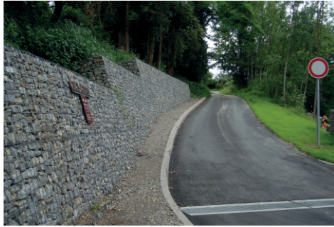
Gabion baskets, made of electro-spot-welded, steel-wire mesh grids
